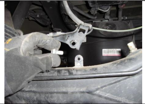
Disconnect ABS wiring brackets from axle.
